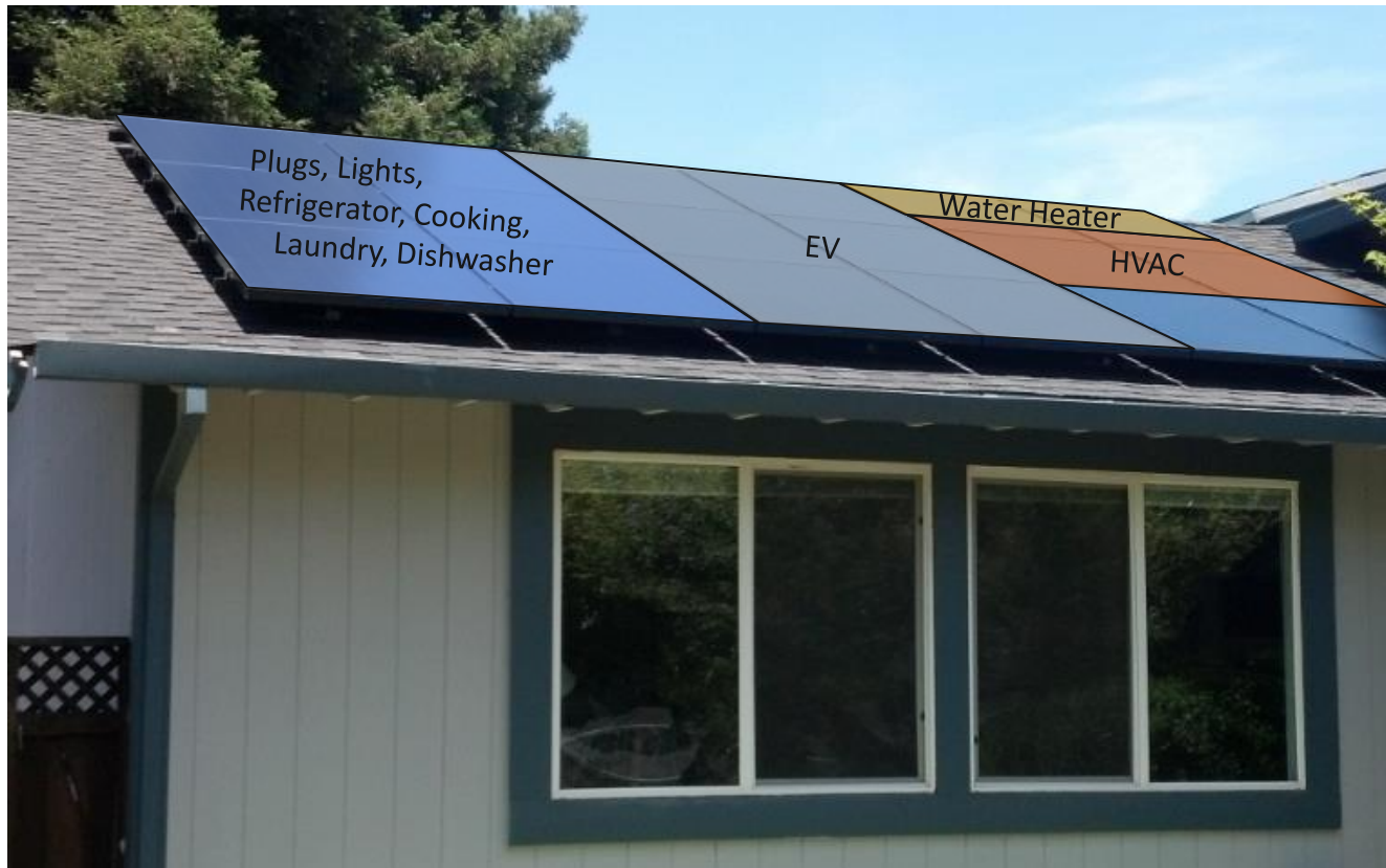
35 year old, 3,000 ft 2 House in Napa, CA after installation of SunPower 6 kW-DC PV System
