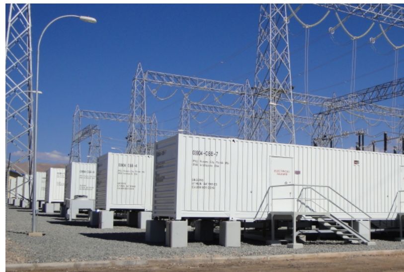
A123 batteries in distribution system
